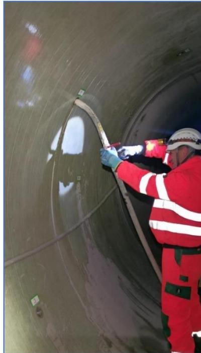
Figure 13. Grout injection phase through valves
