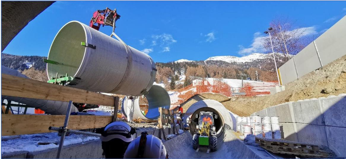
Figure 7. Transport and insertion of GRP pipes in tunnels
