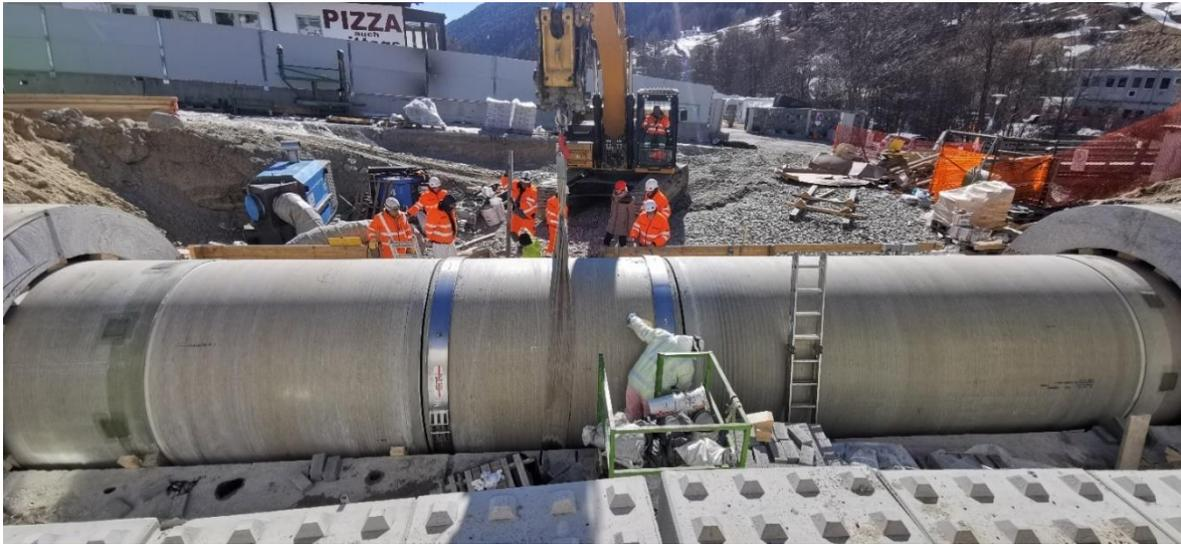
Figure 9. Joint connection system STRAUB OPEN FLEX3 – Last GRP piece
