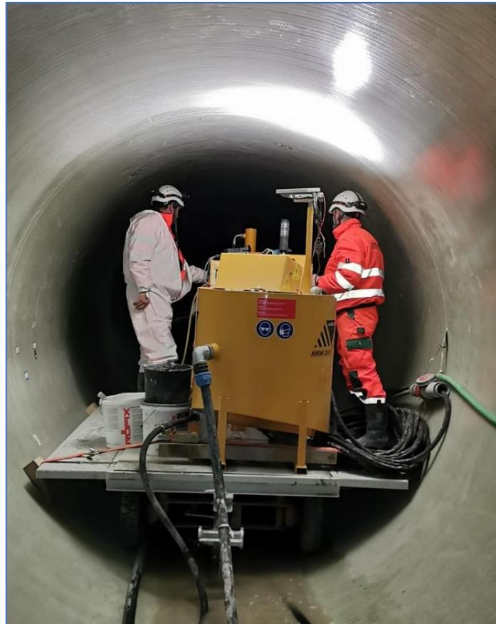
Figure 12. Mortar injection system
