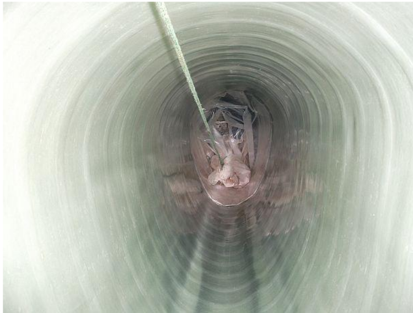
Figure 12: Smooth liner surface after removal of inner film
