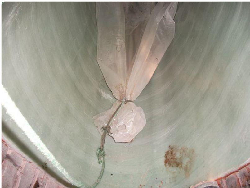
Figure 11: pulling of the inner film
